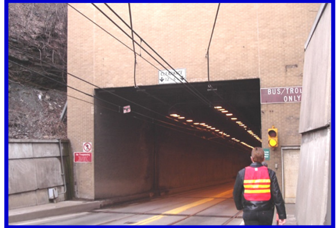
Pittsburg – Mt. Washington Tunnel Portal
